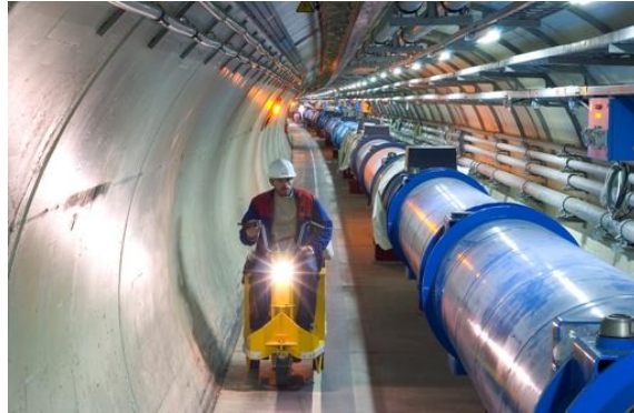
Figure 1: The LHC Tunnel
